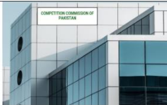
CCP aims to construct a STATE-OF-THE-ART HEADQUARTER in Islamabad
